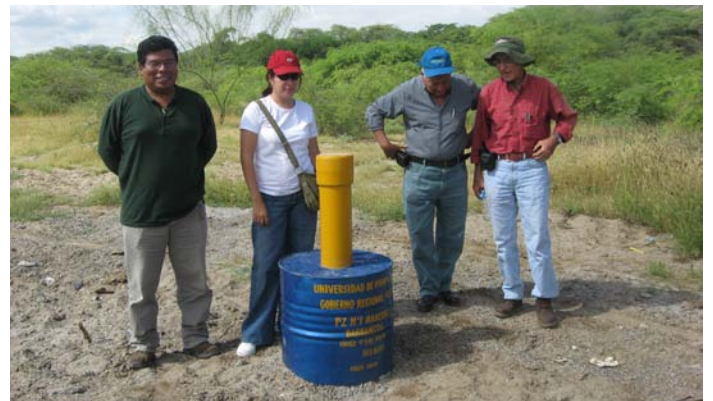
A new 100 m deep piezometer, installed with financial support of the Piura regional government. (Photo credit: T. Vitvar).
